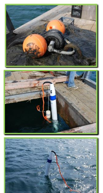
Photo left: The Hazelett Marine conservation mooring system is attached to the anchor block and is ready to be lowered to the bottom. Notice the gooey black and brown sludge on top of the anchor block. Traditional mooring chains must raise a potent cloud of this silt when they drag across the sea bottom.
